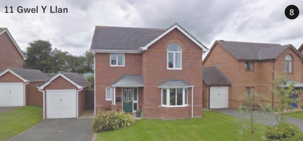
Brics, ffenestr fwaog, ffenestr fae, to llechi
