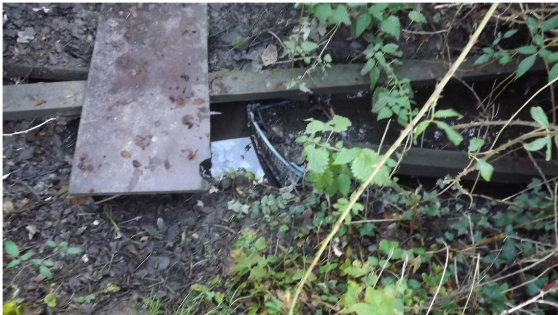
Figure 3.2: an indication of the depth of water
