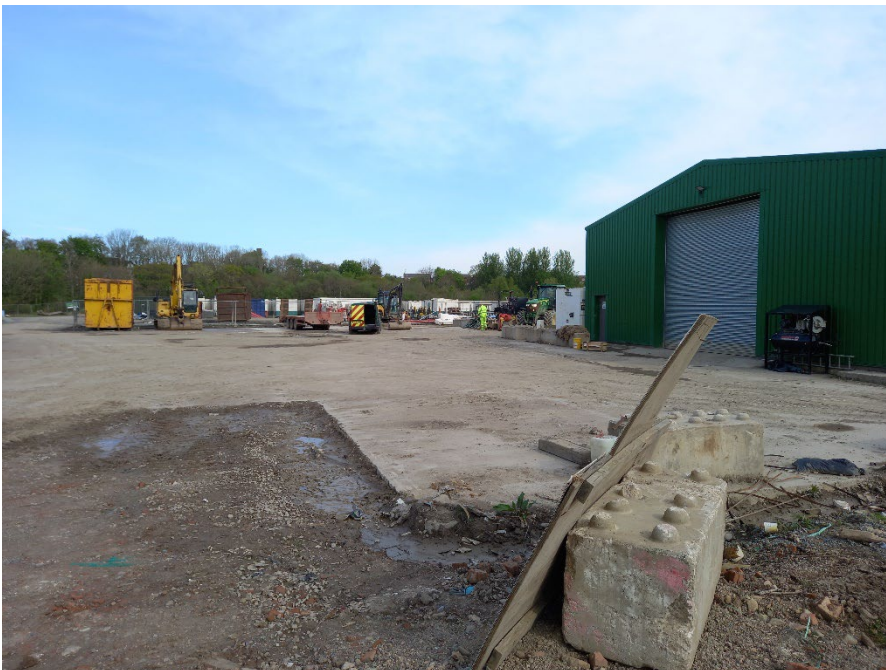
Plant workshop and maintenance area
