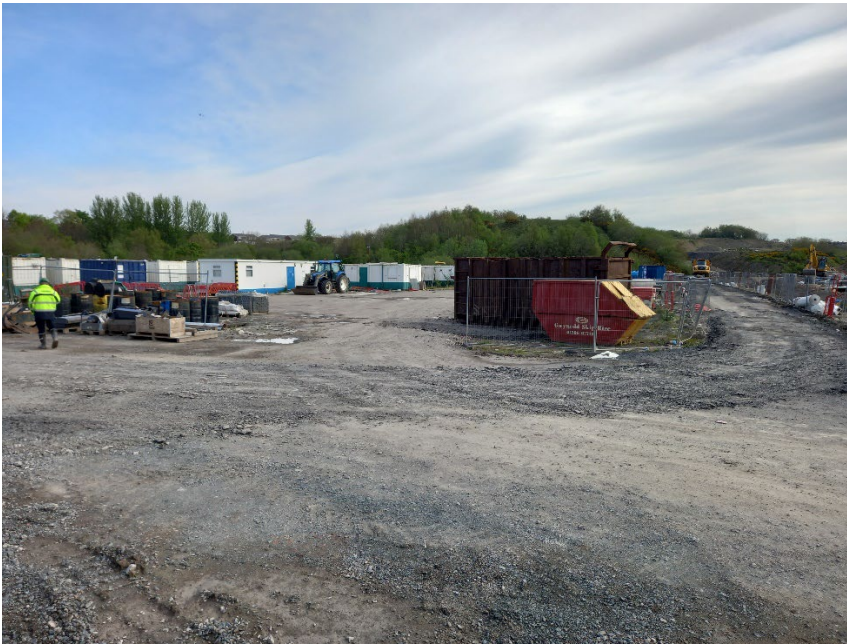
Open storage area at rear of temporary offices
