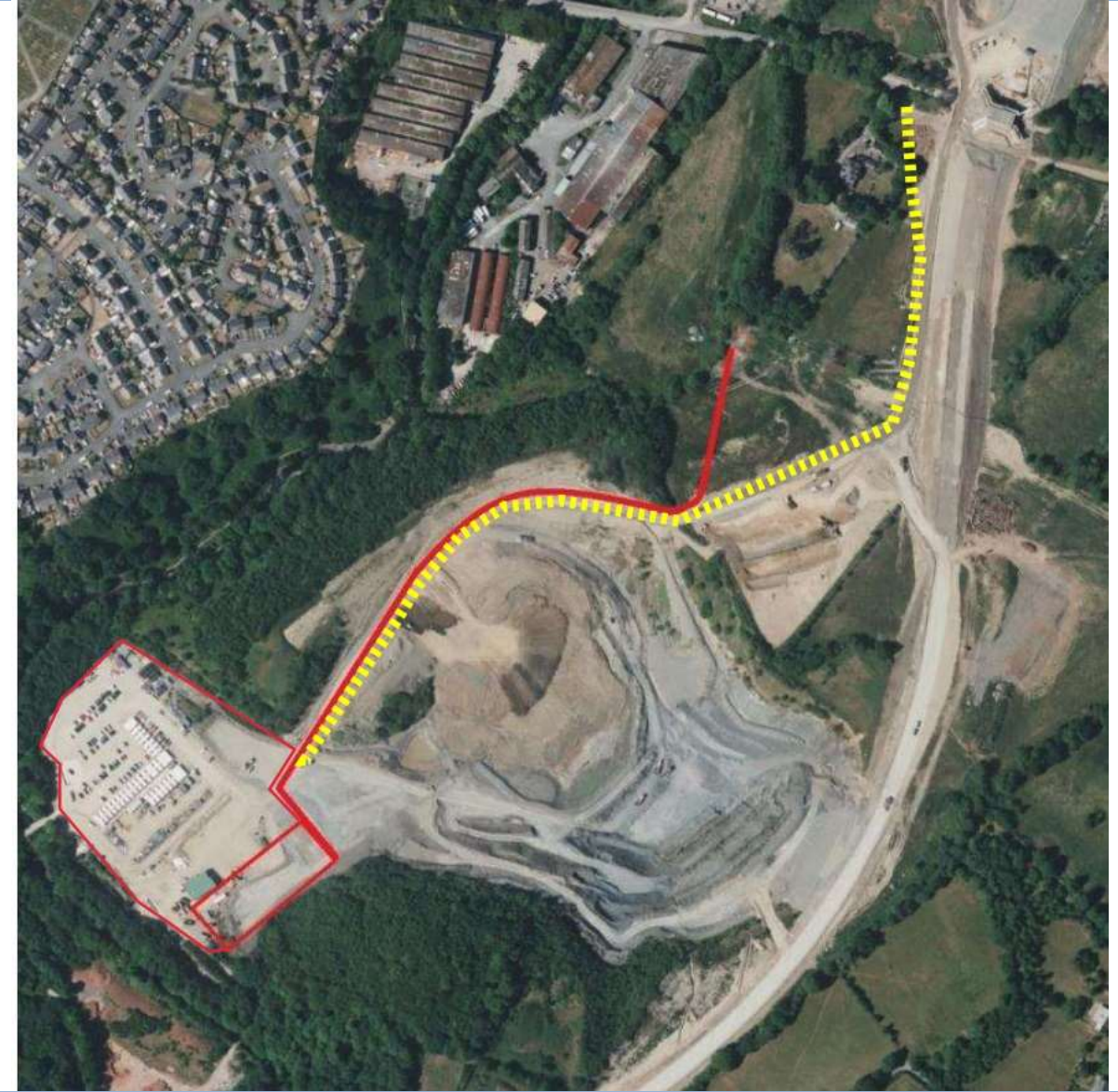
Location of the Peaking plant. Red line shows route of buried services also included in the application.
