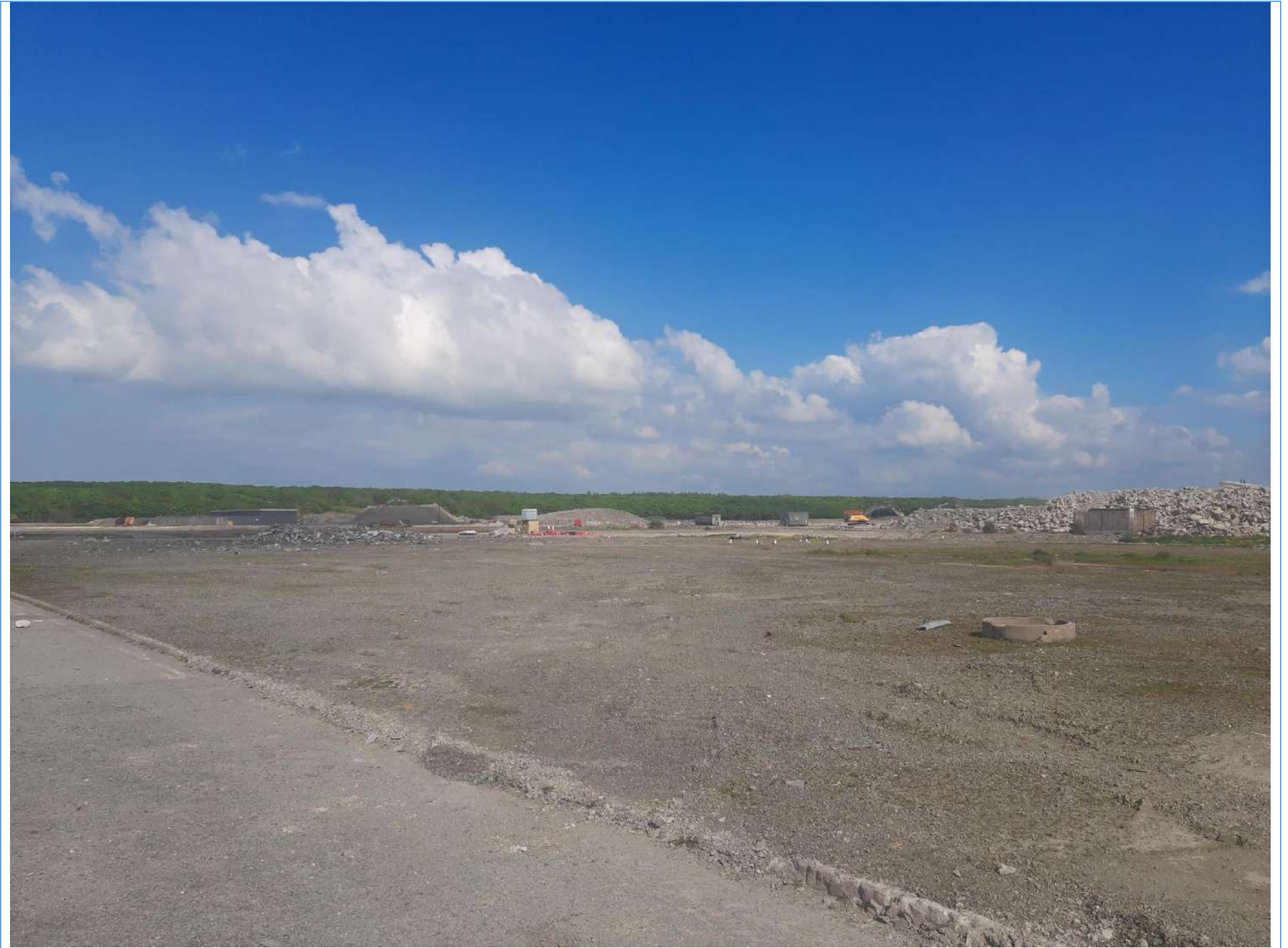
View across the Application Site facing the Northeast boundary.
