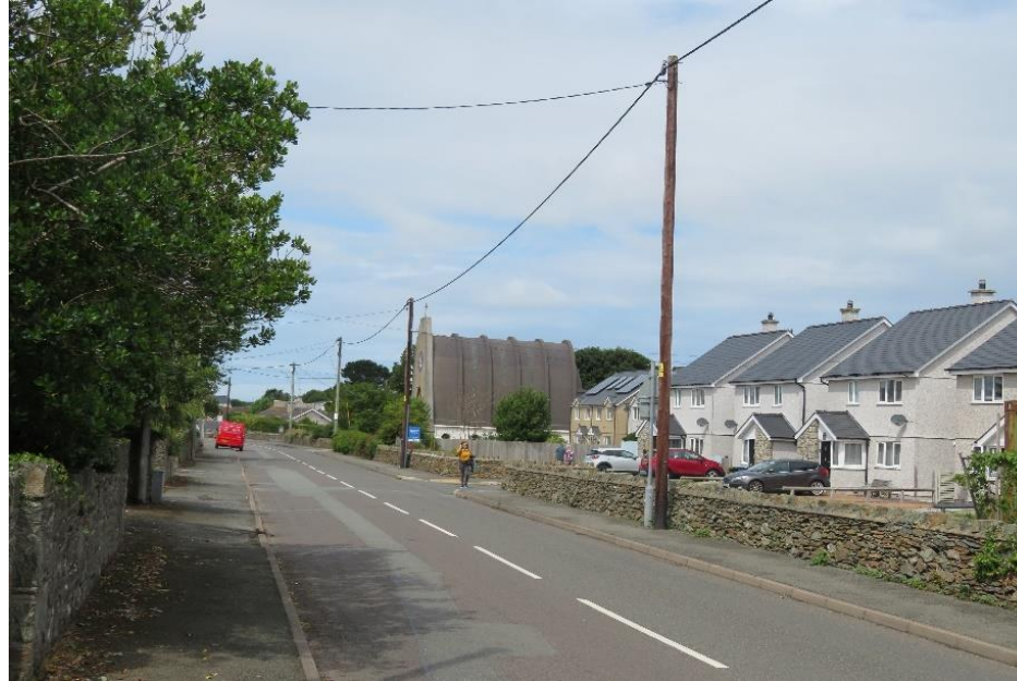
The listed Catholic church from the east with the modern development of houses on the north side of Bull Bay Road in the foreground right.
