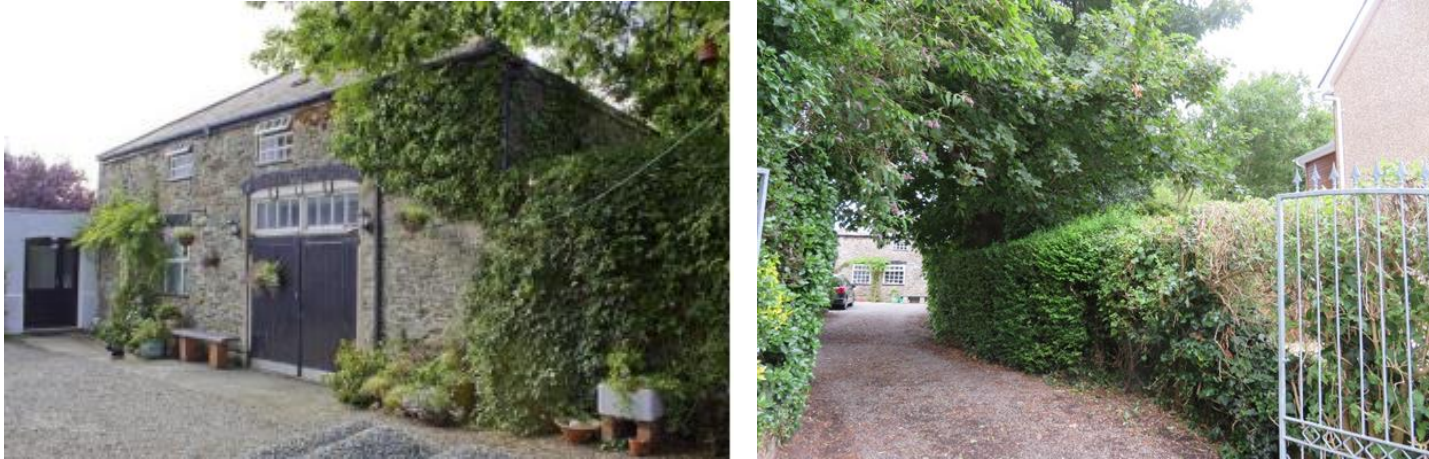
Left: Former Stables to Mona Lodge. The south facing elevation. Right: Glimpse of the former Mona Lodge Stables up the approach drive from Stryd Mona.
