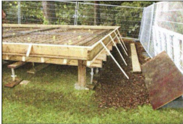
Photo 36: Small diameter piles (less than 150mm) are an effective means of supporting structures in RPAs with minimal disturbance and allow air and water to reach the soil and roots below.
