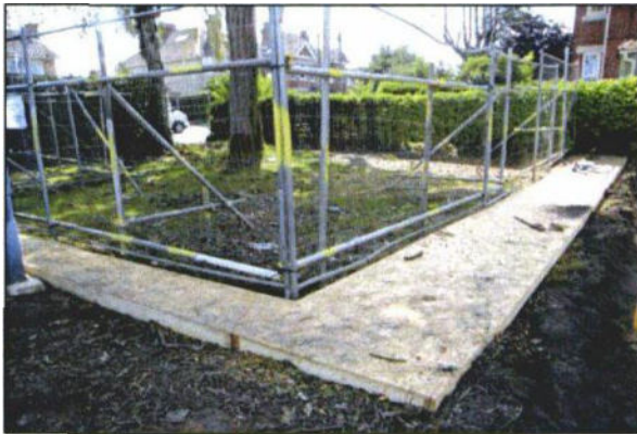
Photo 9: Plywood fixed to a wood frame is another effective method of protecting soil from pedestrian compaction.
