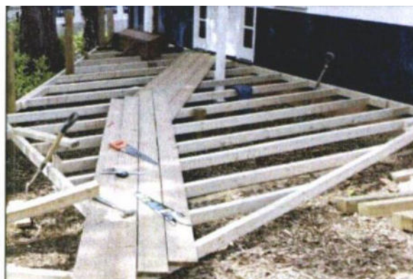
Photo 35: This deck supported above the ground on small posts provides a low-impact alternative to conventional stone patio surfacing in RPAs.
