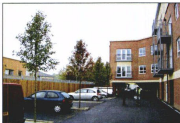
Photo 54: It allows trees to be successfully established in areas of extensive hard surfacing, with very little, if any, loss of parking space.
