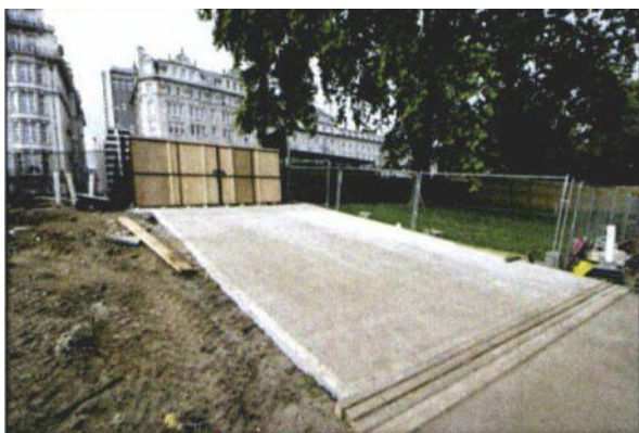
Photo 30: This temporary access for heavy construction traffic on the outer edge of a RPA is a concrete slab cast above ground level and will be removed when the project is completed.
