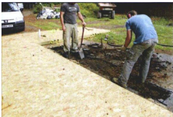
Photo 15: Careful hand-digging using conventional tools is acceptable for exposing roots in RPAs.
