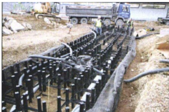
Photo 55: The individual Silva Cells can be assembled in layers and service ducting threaded through before filling with soil and fitting the reinforced tops.
