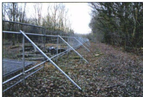
Photo 2: Heras fencing wired to scaffold braced posts is a robust and effective interpretation of the BS specification.
