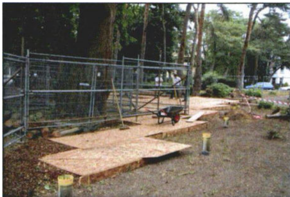
Photo 40: Once the piles have been installed (yellow tops), the ground protection to support the piling rig is removed ready to fix the void-former onto the bare soil, in advance of pouring the building slab.
