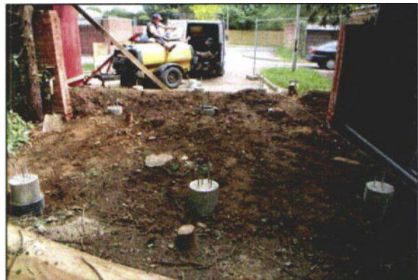
Photo 41: Piles can also be used to support bridges across sensitive RPAs, but the temporary ground protection has to be removed before the main structure is either imported in or cast on site.
