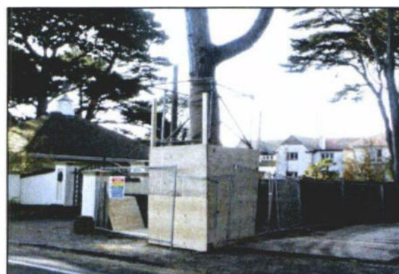
Photo 6: Board secured to scaffold framework adds another layer of protection for vulnerable trunks and branches.
