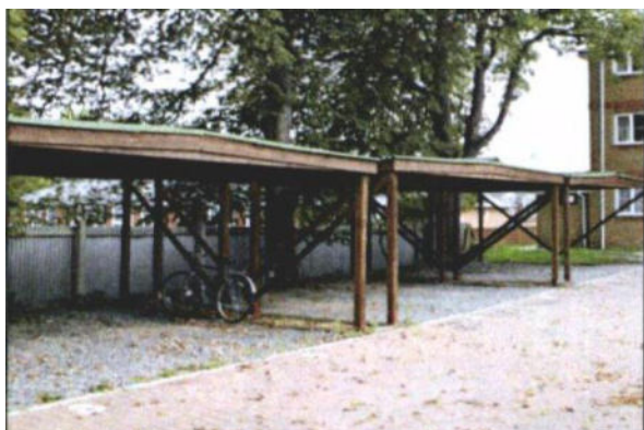
Photo 34: These carports are formed by wooden posts above a three dimensional cellular no-dig and load-spreading surface of permeable crushed stone.
