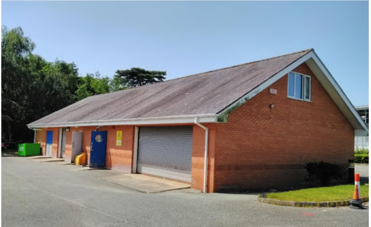
Photo of the existing Llyn Brain Annexe building illustrating the roller shutter access to the workshop and gable end window to the first-floor accommodation.
