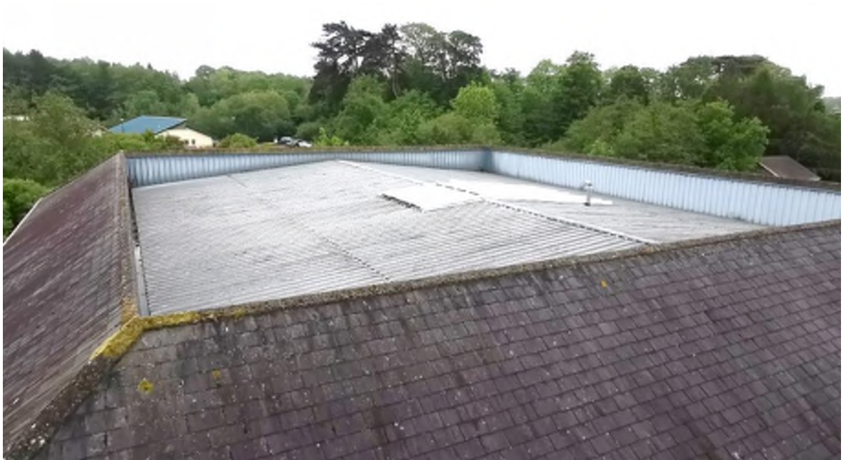
Photo of the existing Llwyn Brain roof.
