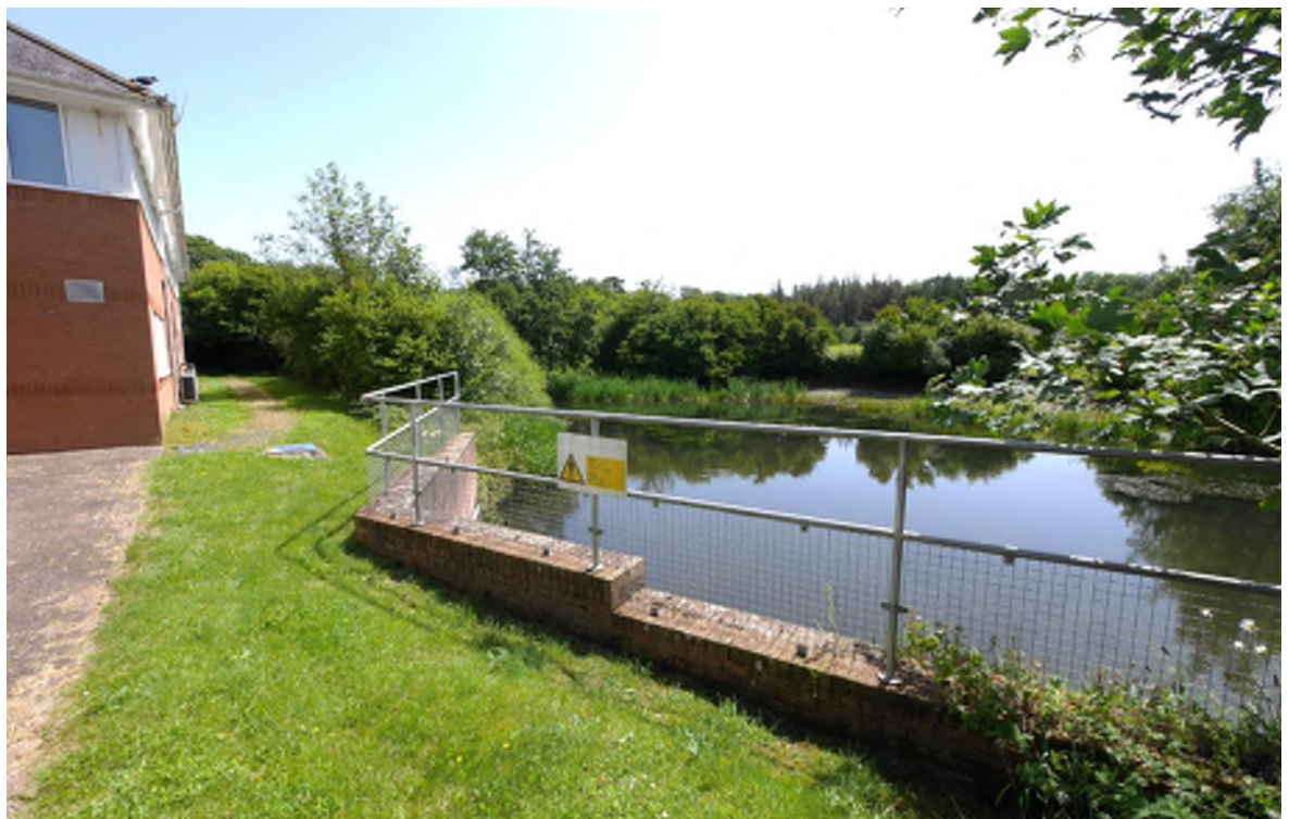
Photo of the existing Llwyn Brain building rear elevation overlooking the neighbouring pond.
