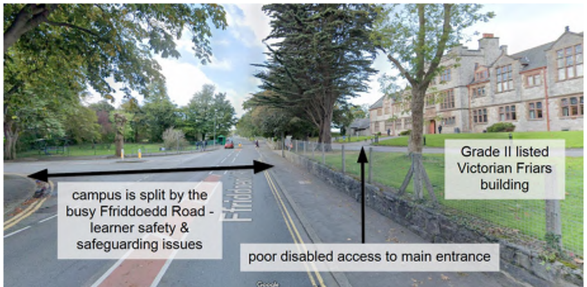
Photo looking down Ffriddoedd Road showing the Friars building frontage & entrance.
