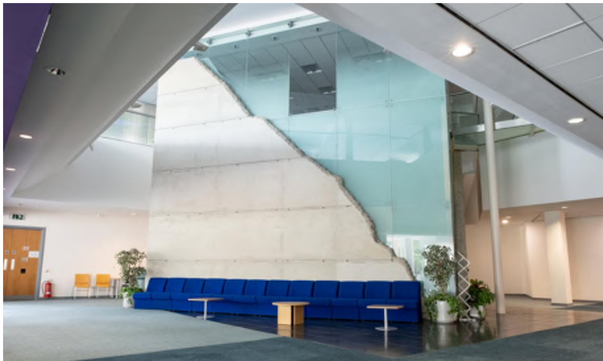
Photo of the existing 'cube' structure and floor void, as seen from the ground floor canteen servery.
