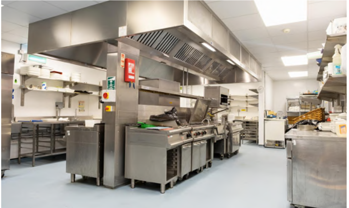
Photo of the existing catering kitchen.
