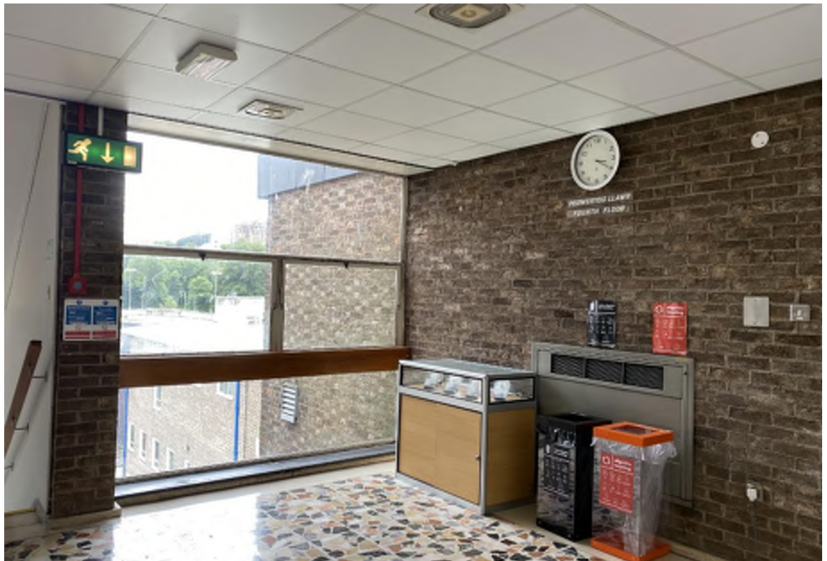
Photo of the engineering block central stair core, fourth floor (third on GA plans) showing single glazed uninsulated Crittal-type metal framed window system (indicative throughout).
