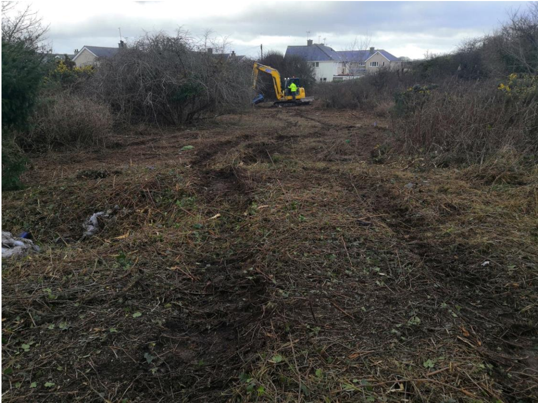
An area of the site following clearance works
