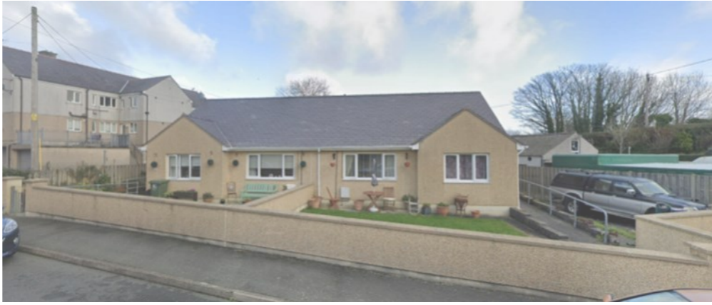
Bethesda St - Pebbledash, facing gables, slate roof
