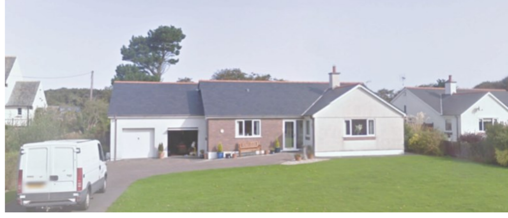
Bull Bay Rd - Brick and pebbledash, facing gable, slate roof
