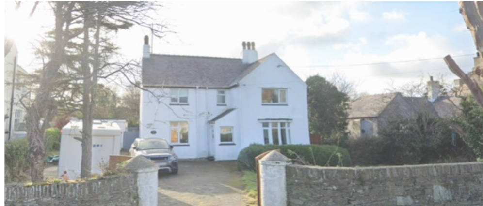
Bull Bay Rd - White render, slate roof , gable front
