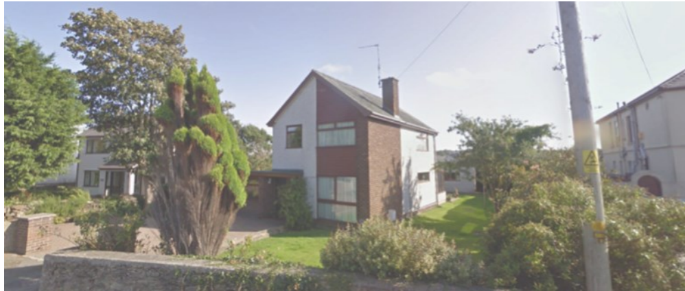
Bull Bay Rd - Half brick and render gable, slate roof
