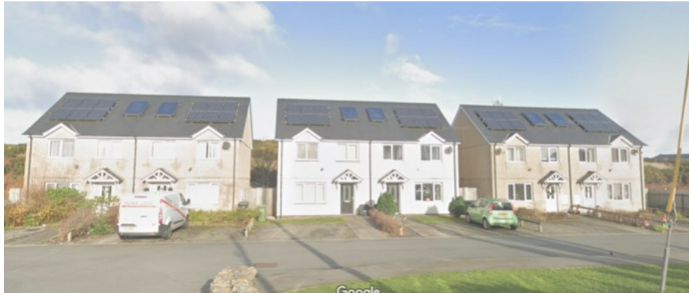
Bull Bay Rd - Pebbledash, door canopies, slate roofs, solar panelling
