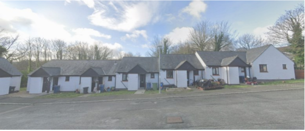
Trehinon - White render, brick cills and heads, slate roof
