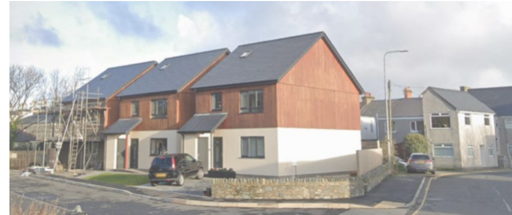
Bull Bay Rd - White render, timber cladding, door canopies, slate roof
