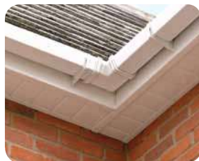
9mm hollow soffit detail
