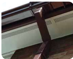
9mm foam soffit detail
